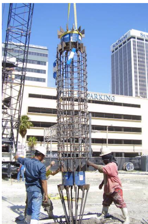
Assembly of a multi-level O-cell arrangement
