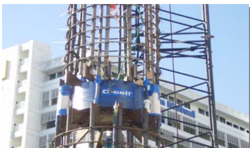
CFA test pile O-cell assembly ready for placement
