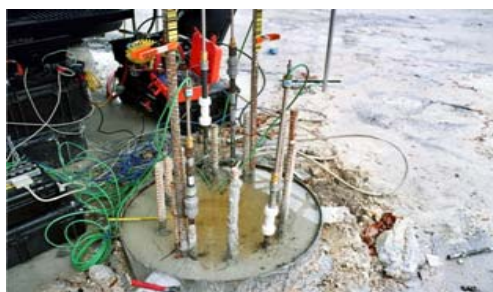
+20 MN CFA test in progress
